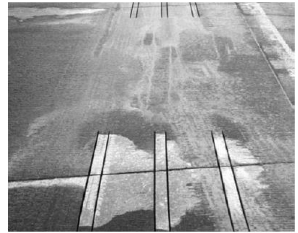
Figure 2.3. Dowel bar slots cut using a diamond-bladed slow cutting machine across a skewed joint (note that the slots are parallel to the centerline and not perpendicular to the joint).
