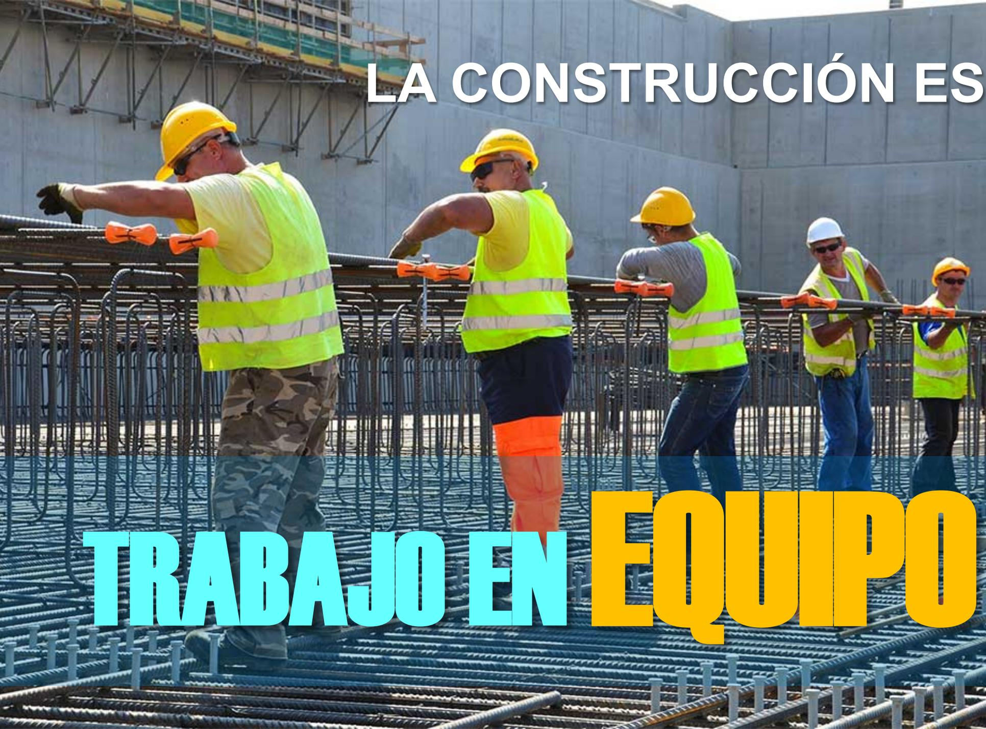
A photograph of five construction workers on a building site. They are standing on a grid of steel reinforcement bars (rebar) laid out on a concrete slab. The workers are wearing safety gear: yellow hard hats, high-visibility yellow safety vests with reflective stripes, and safety glasses. They are using orange-handled tools to work with the rebar. In the background, there are concrete walls and scaffolding. The scene is brightly lit, suggesting a sunny day.
