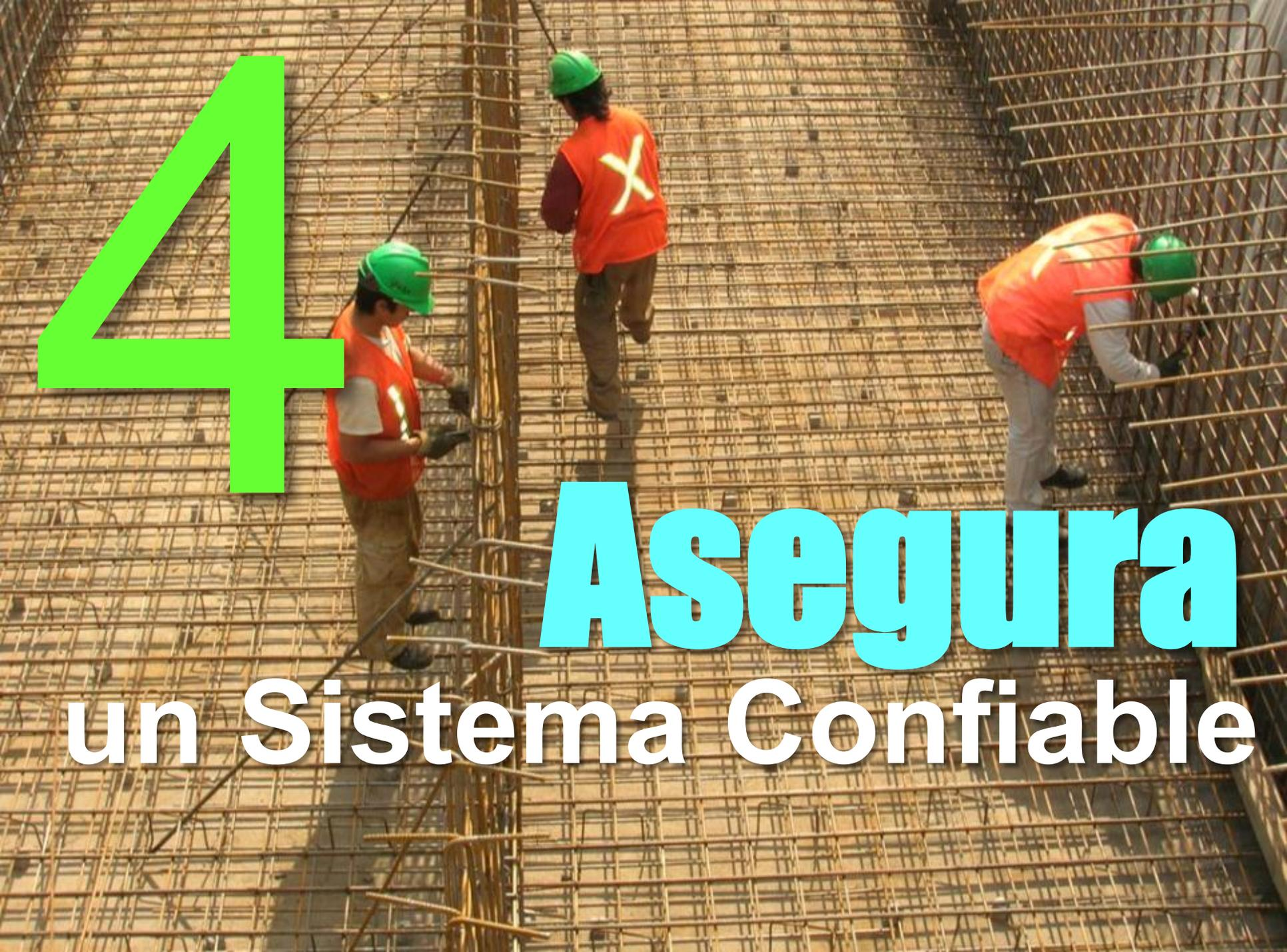
A high-angle photograph of three construction workers on a large-scale rebar grid. The workers are wearing orange safety vests and green hard hats. One worker in the center has a white 'X' on their vest. They are surrounded by a dense network of steel reinforcement bars (rebar) laid out on a wooden formwork. The scene is brightly lit, suggesting an outdoor or well-lit indoor construction site.
